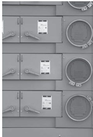
FSMC Units Installed in Pow-R-Line C Switchboard
