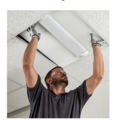
With its low-profile design, the BLT offers greater installation flexibility, especially in applications where plenum space is limited.
